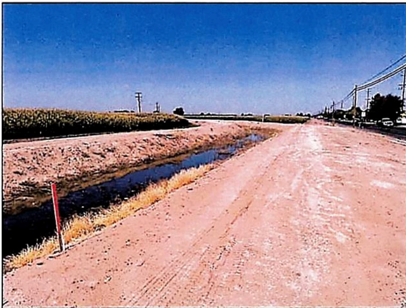
View looking west along the ROW and TCE take areas from the northeast corner of the property near the street intersection.
